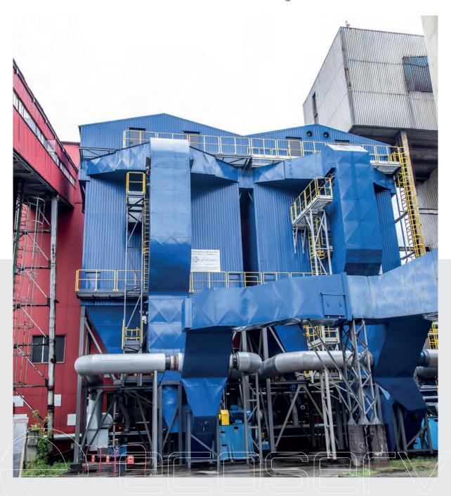
compressed air occurs cyclically (the time between compressed air pulses is set) or automatically (when the differential pressure exceeds the set value in the filter controller).
